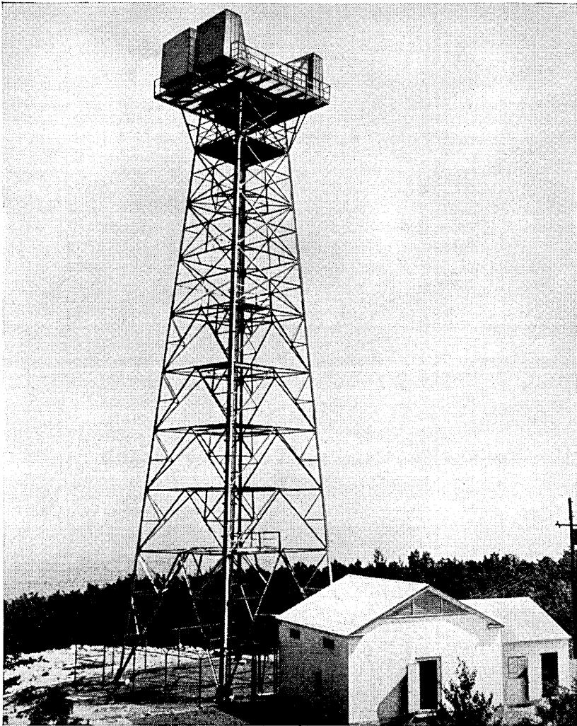
FIG. 10—Microwave radio relay tower at Cotoctin Mountain, Maryland, on a New York-Washington radio route. There are 300 message circuits in service with more planned.
