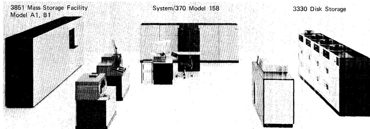
Figure 7-71. IBM 3850 Mass Storage System with 3851 Mass Storage Facility, System/370 Model 158, and 3330 Disk Storage
